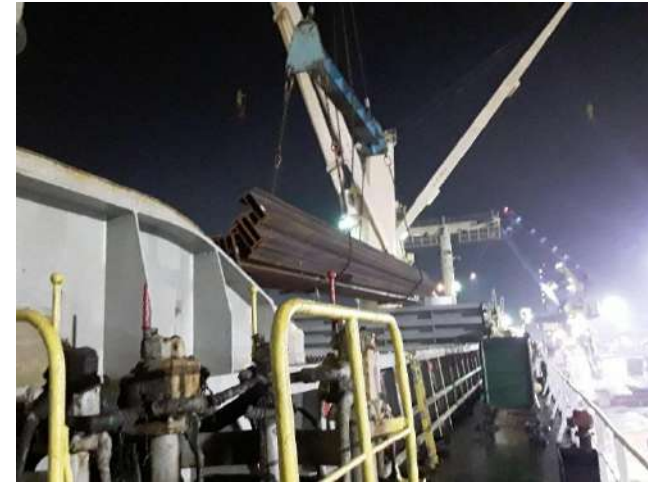
Basket lift of channels with 2 chains under a spreader bar
