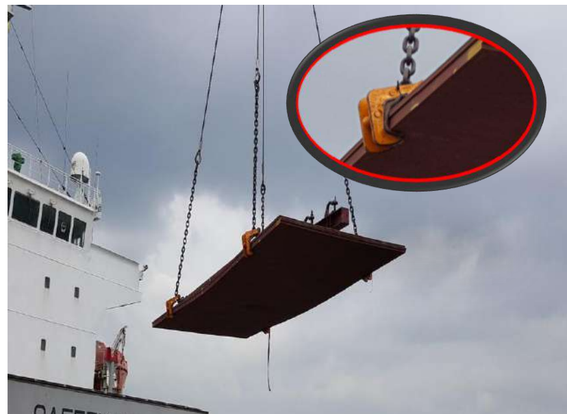
'C' Hooks and a spreader used for off-loading of steel plates.
