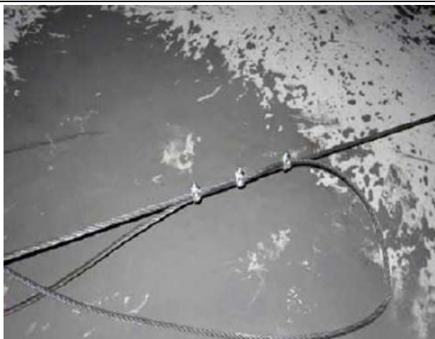
Incorrect use of bulldog grips
