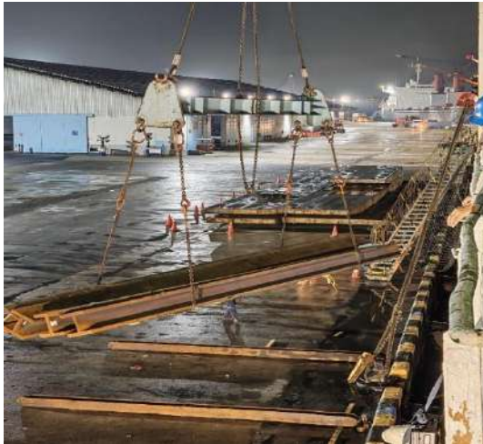
Basket lift of channels with 2 chains under a spreader bar
