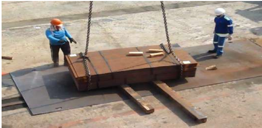
Bundled steel plates ready for loading. Choke hitch chain sling in use.
