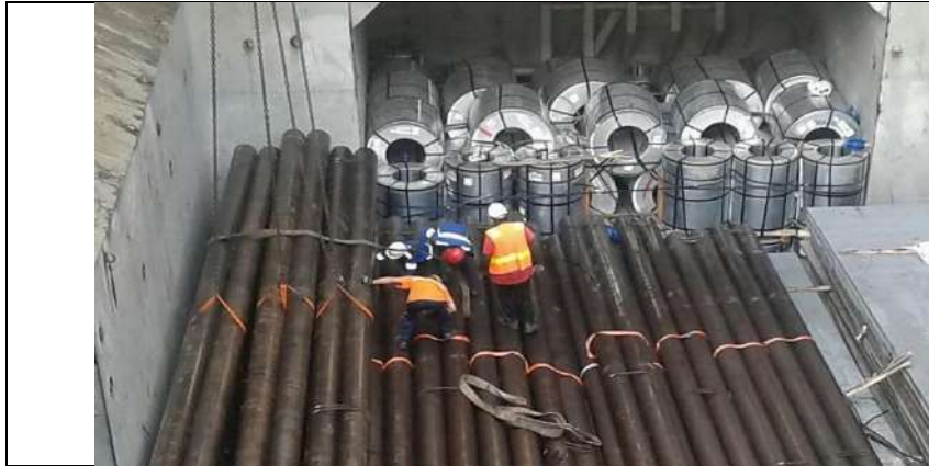
Pre-slung pipes being discharged.
