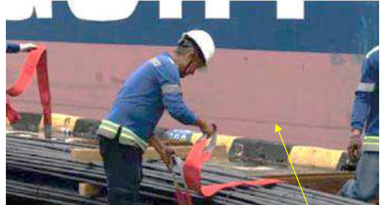
Pre-slinging of two tiers of rebar in preparation for loading.
