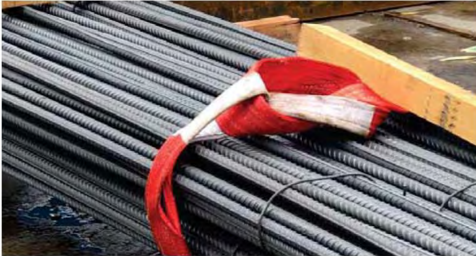
✔ A sling combining 6 bundles of rebar ready for loading
