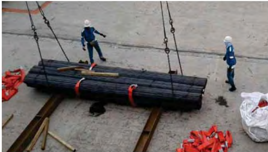
✔ Pre-slung 6 m long bundles about to be loaded. Pre-slinging reduces the time needed for discharge operations
