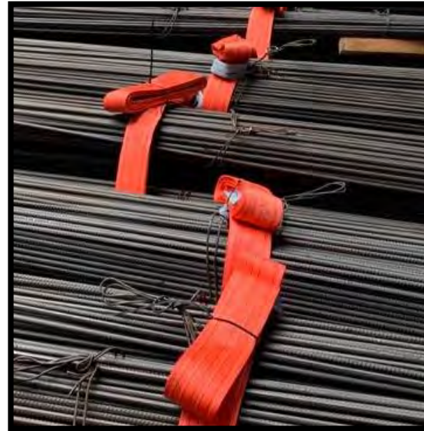
Sling secured tight with zip ties with eyes on top during loading so that riggers at discharge port can access easily.
