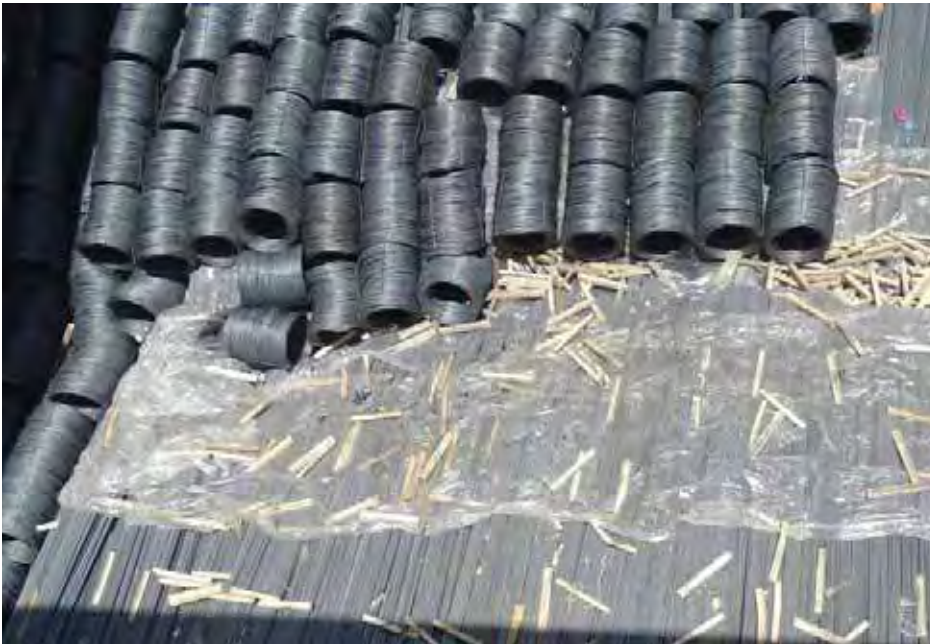
WRIC loaded on top of rebar, segregated with plastic sheets
