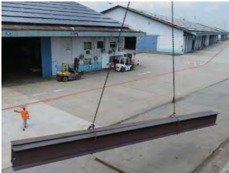
An application of the two-leg chain choke hitch around the I-beams.
